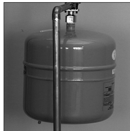
Figure 23: The Thermal Expansion Tank should be pressurized with air, using a hand pump, to match the home's incoming water pressure.
