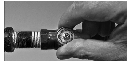
Figure 48: Gas valve in "on" position.
