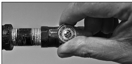
Figure 30: Gas valve in "on" position
