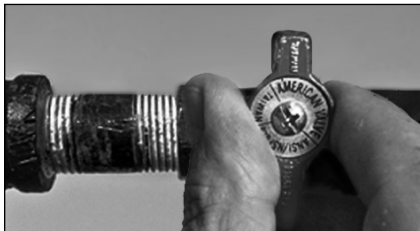
Figure 44: Gas valve in "off" position.
