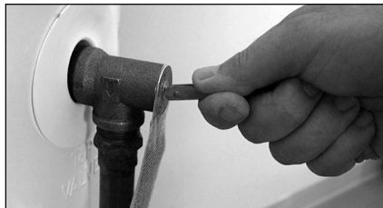
Figure 41: T&P Relief Valve.
