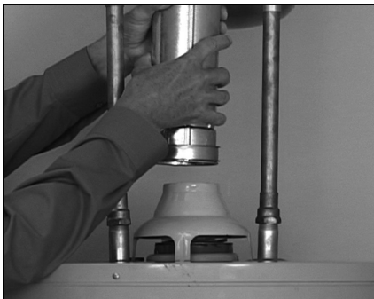
Figure 14: Disconnect the vent pipe (roof jack) from the draft hood.
