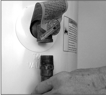
Figure 13: Removing the T&P Relief Valve discharge pipe.
