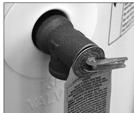
Figure 18: Temperature and Pressure Relief Valve
