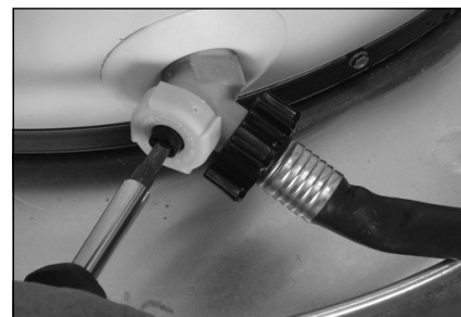
Figure 12: Draining the old water heater.
